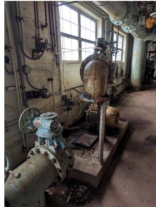
SOFTENER SYSTEM UPFLOW PUMP REPLACEMENT
