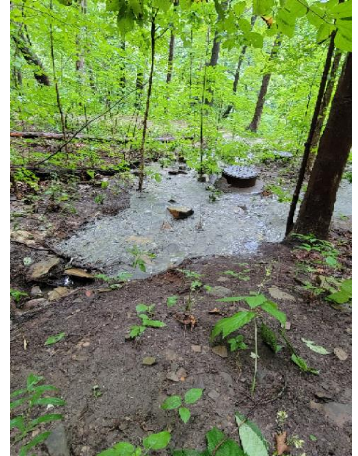
GORGE TRUNK SEWER EMERGENCY REPAIR
