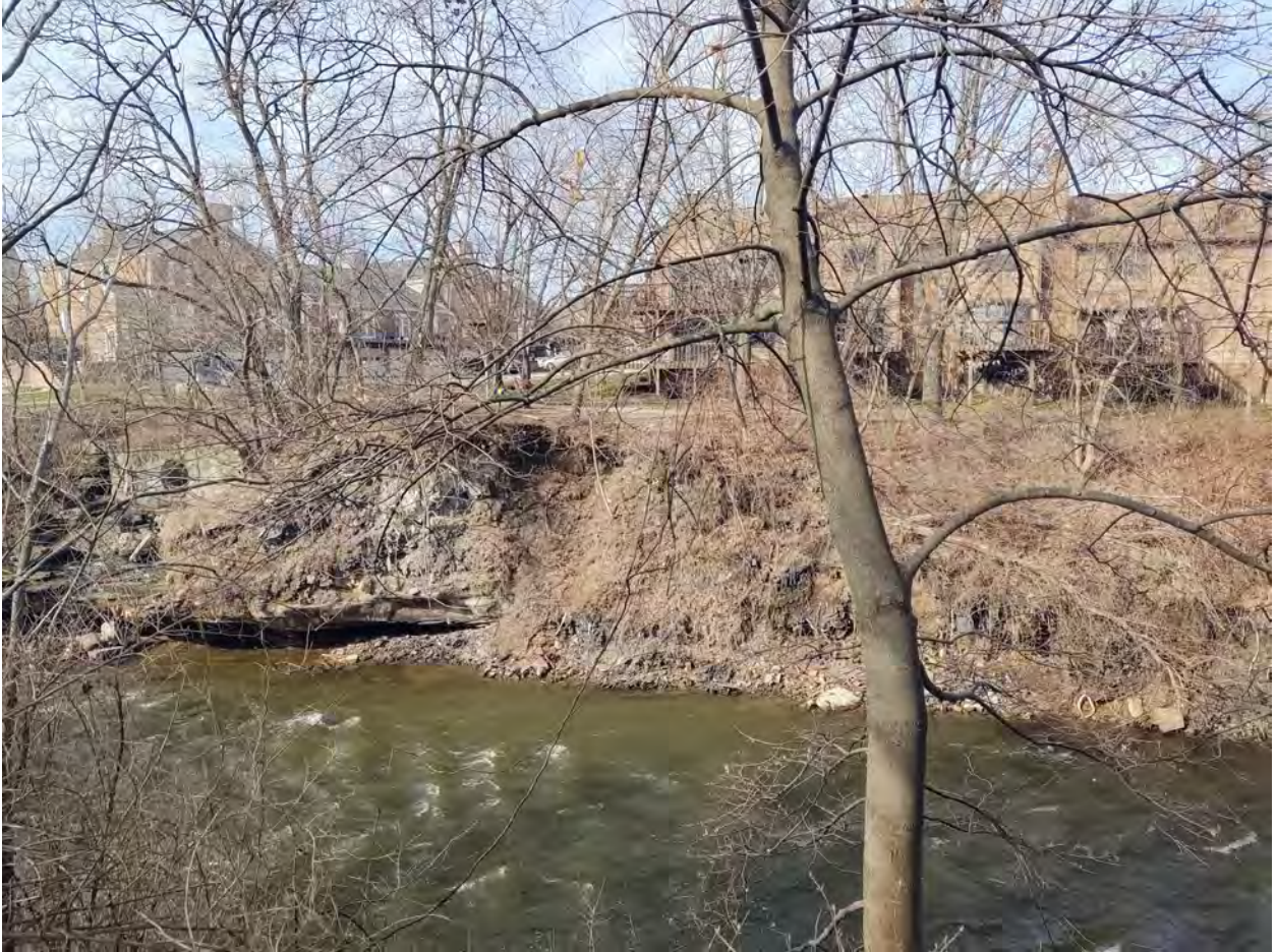
Photo 1. View of project site and severe erosion from across the river.
