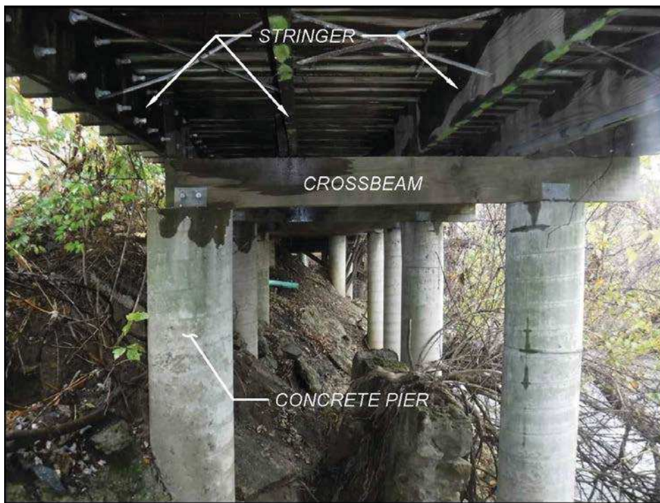
Figure 3 - Section 1 and 2 Timber Boardwalk
