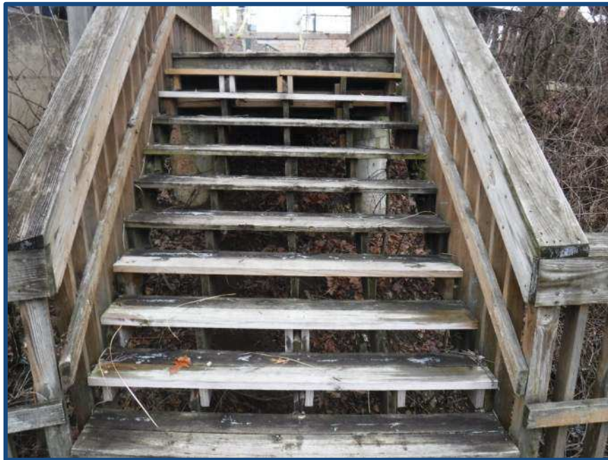
Existing Boardwalk Access Point 'B'
