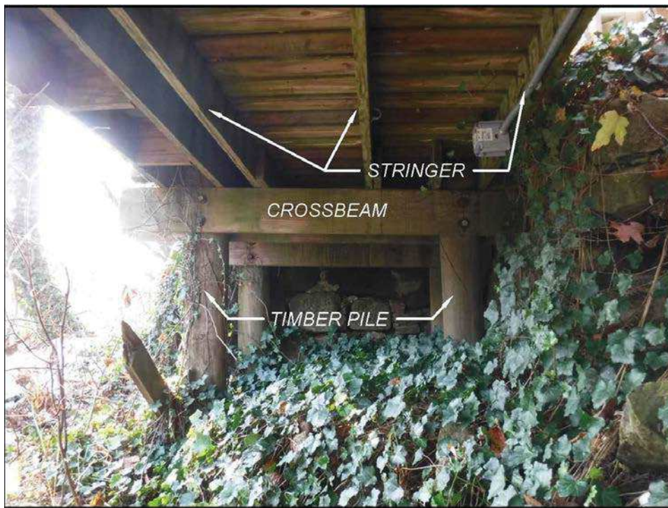
Figure 7 – Section 4 Timber Boardwalk
