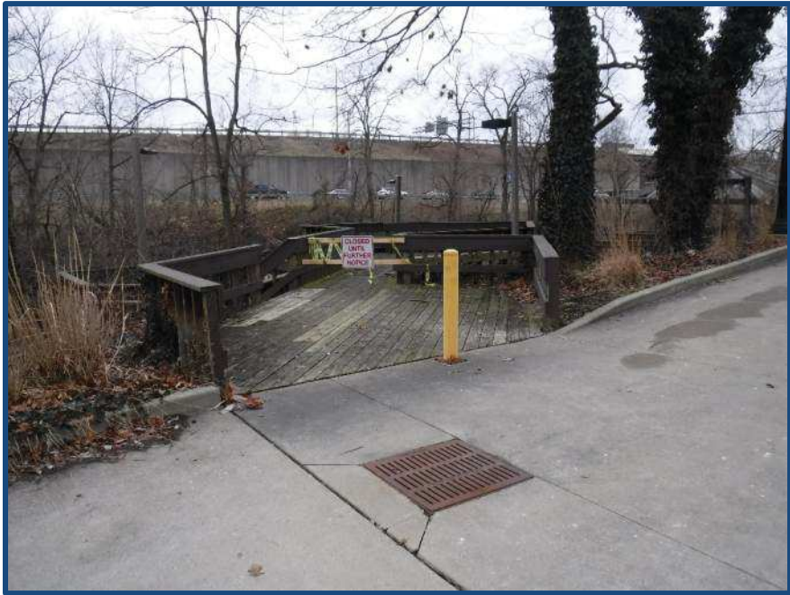
Existing Boardwalk Access Point 'D'
